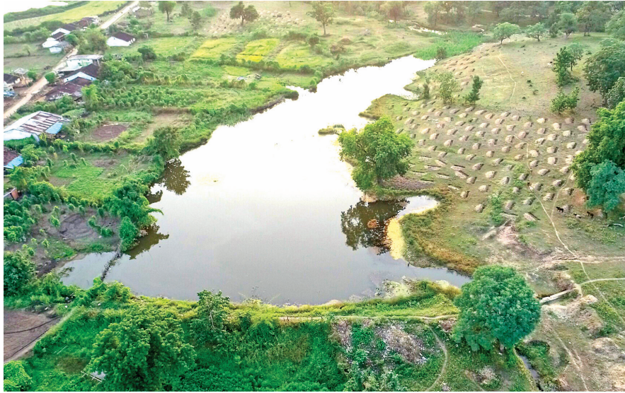
Community-driven water harvesting structure, Itarsi, MP
